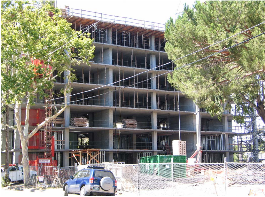
FIGURE 1 ELEVATION OF TAYLOR TOWER UNDER CONSTRUCTION
