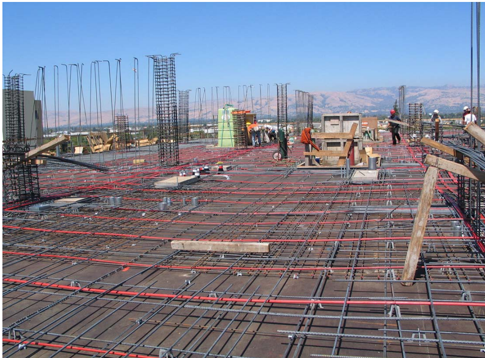
FIGURE 2 TENDON LAYOUT OF ONE OF THE FLOORS
